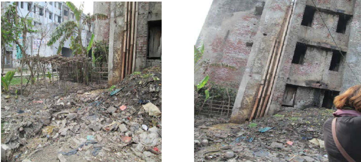
Figure 4: Waste and wastewater including sewage dumping practices before the DEWATS implementation.
